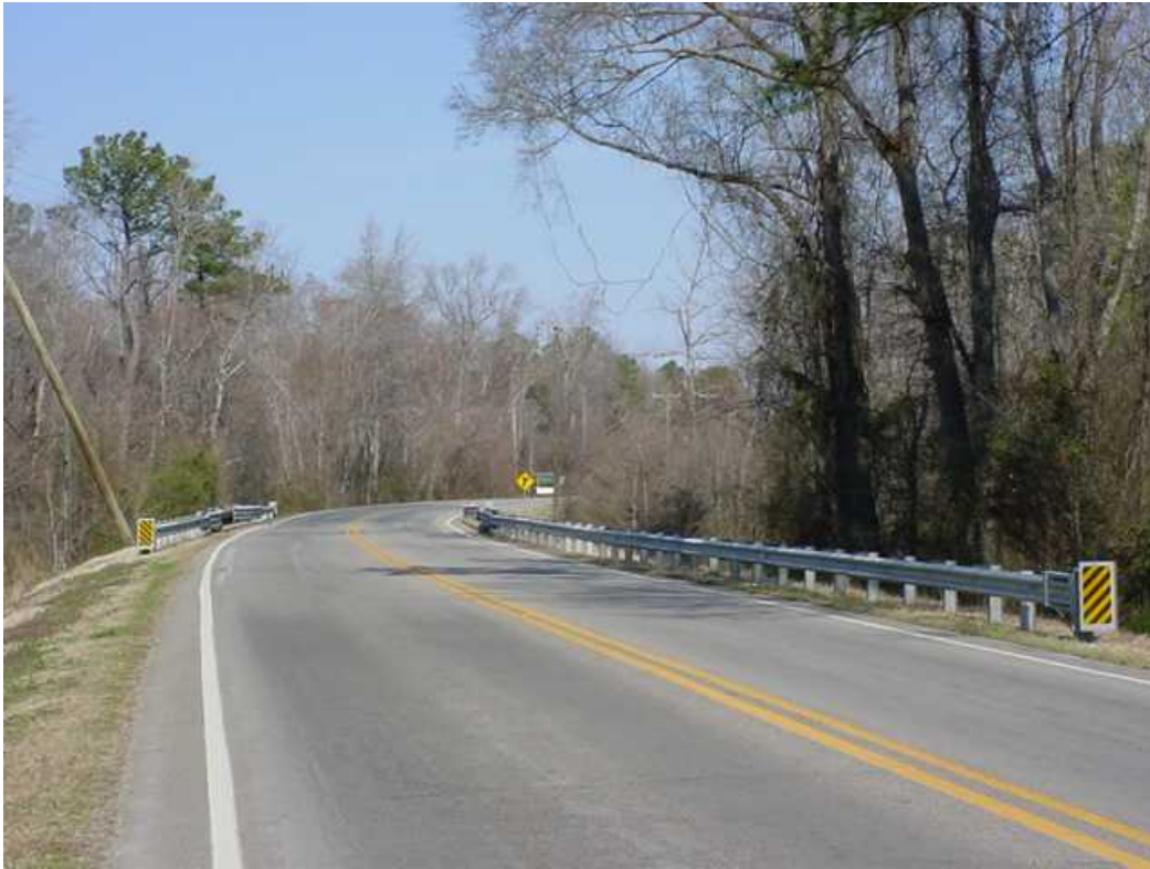
Between Bridge #12 & #25 looking North at Bridge #25
