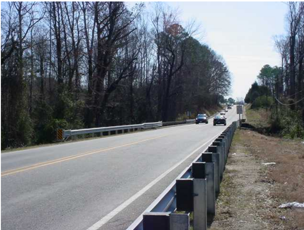
Between Bridge #12 & #25 looking South
