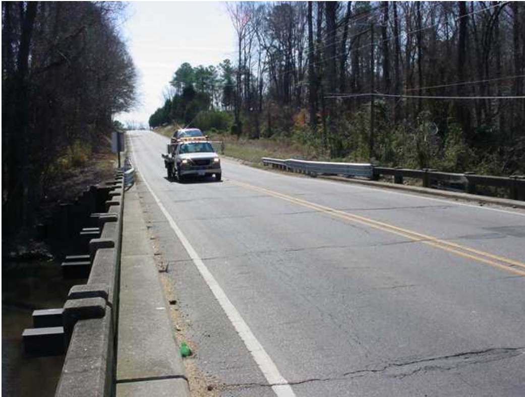
Standing on Bridge #12 looking South
