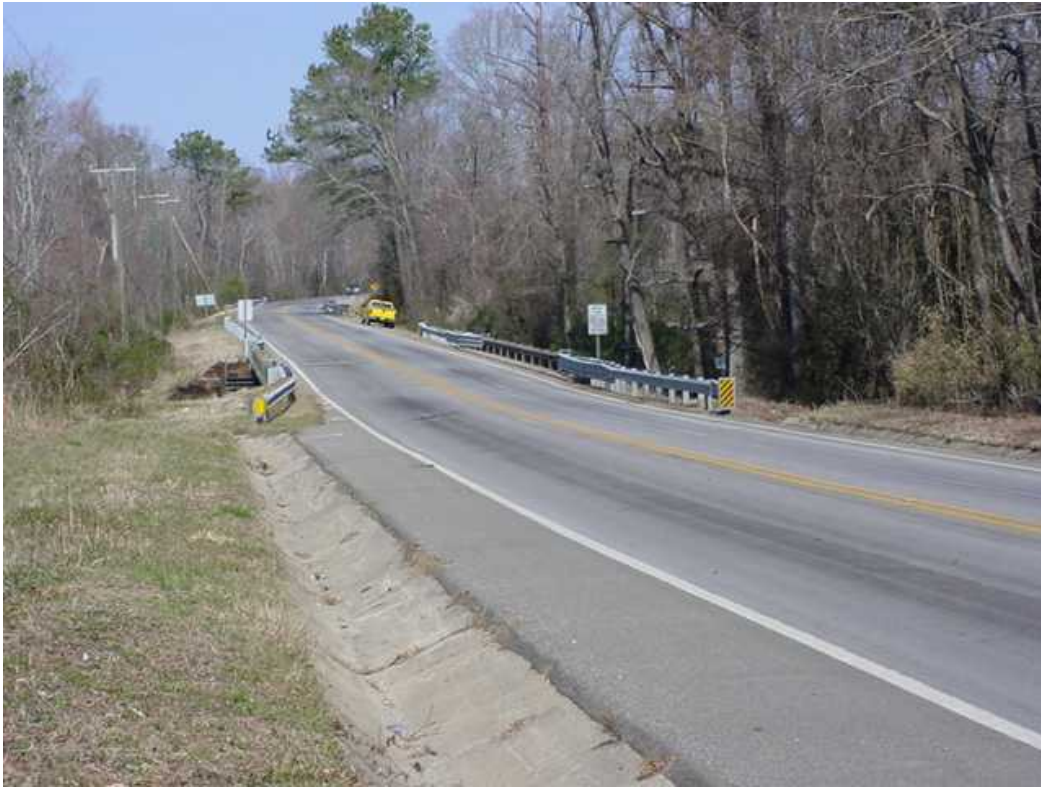
Looking North toward Bridge #12
