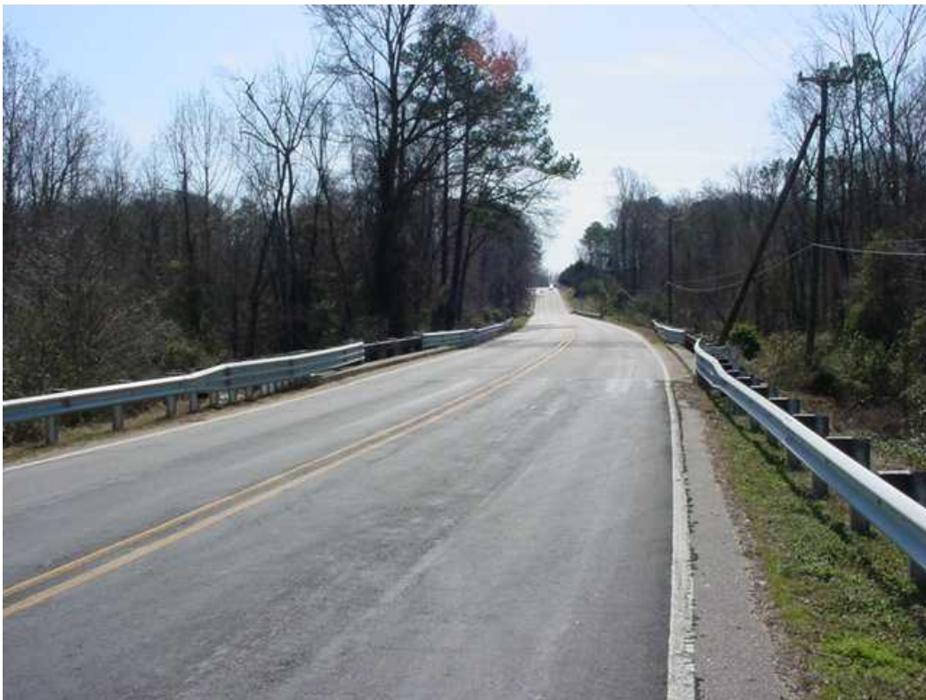
Just North of Bridge #25 looking South
