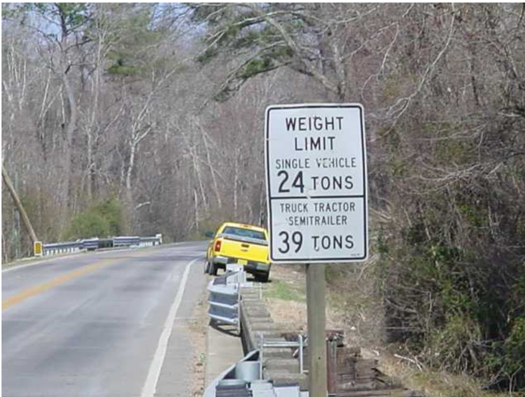
Posting Sign at Bridge #12
