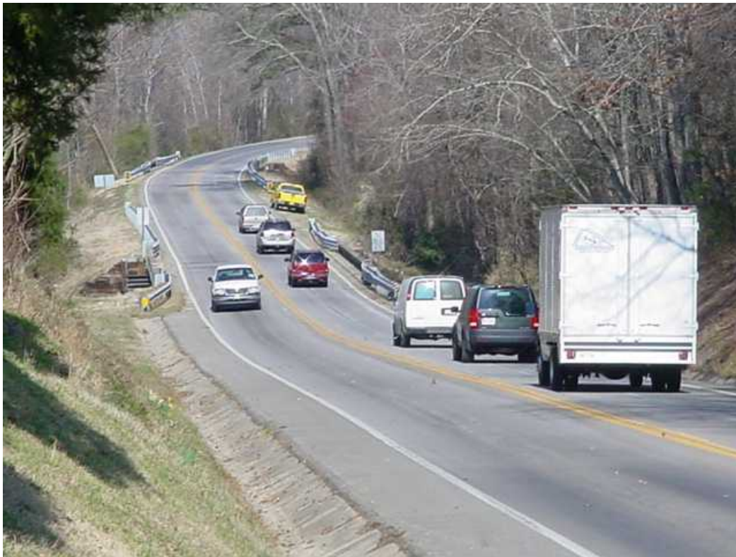
Looking North toward Bridge #12
