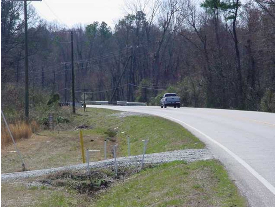
North of Bridge #25 looking South at Private Drive
